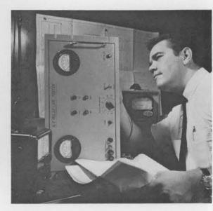
CHECKING OUT a relay life tester built by electronics apprentices, James Lujan (4233-2) uses a volt-ohmmeter. In addition to their study of the theory and assembly of electronic equipment, apprentices learn to operate a variety of electronics test equipment, and to interpret test results. A Sandian for six years, Jim came to the program from Sandia Laboratory's Printing Section.
